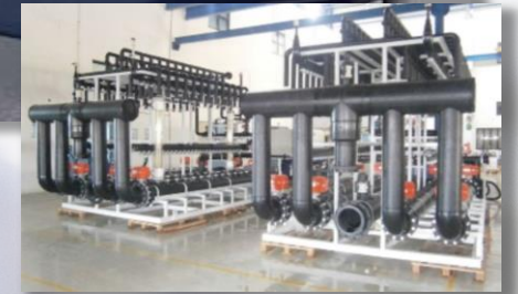
Pontoon Data Center
